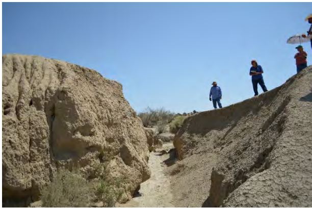
A breached earthen dam in Huerfano community that was once a source of water for wildlife and livestock. There is a need for standardize engineering designs for earthen dams across the Navajo Nation.
